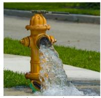
the growth of microorganisms within distribution mains. Flushing helps remove stale water and ensures the presence of fresh water with sufficient dissolved oxygen, disinfectant levels, and an acceptable taste and smell.
